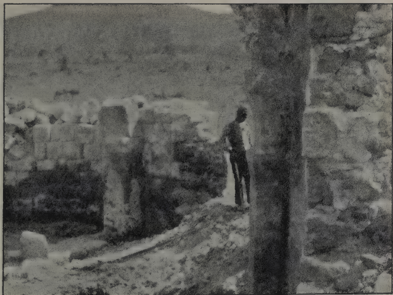
FIG. 67.—No. 10, interior, showing engaged columns on either side of W. door.
